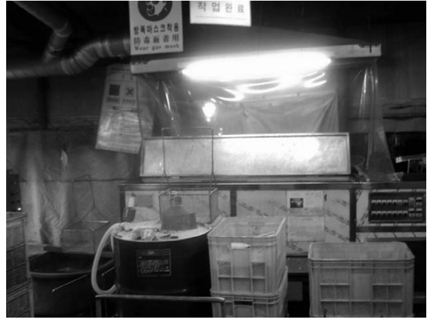
Fig. 2. Degreasing bath & local exhaust ventilation hood in the factory.
