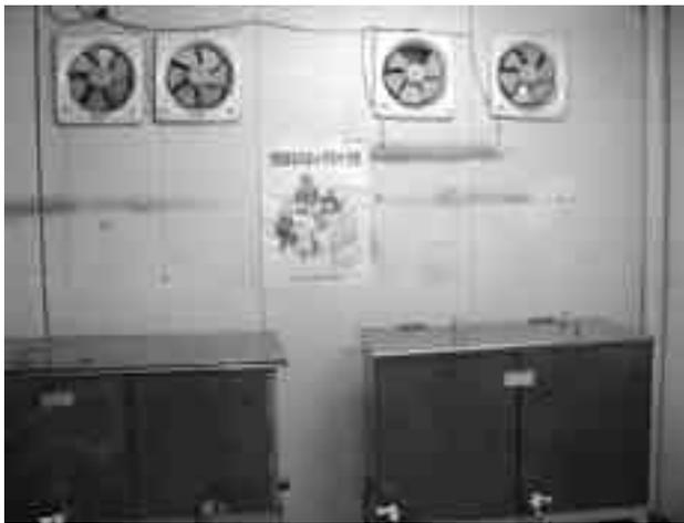
**Fig. 1.** Ventilation system in the workplace and cleansing boxes filled with n-hexane
